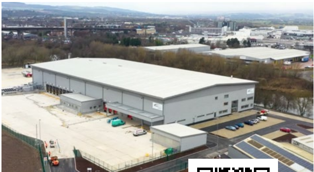
View our video Temperature Controlled Storage Facility in Glasgow
